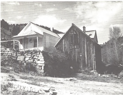
FIGURE 2-33. Old Ice Building (Block 7, Lot 31). This building has been moved and attached to the building next door (Block 7, Lot 32).
